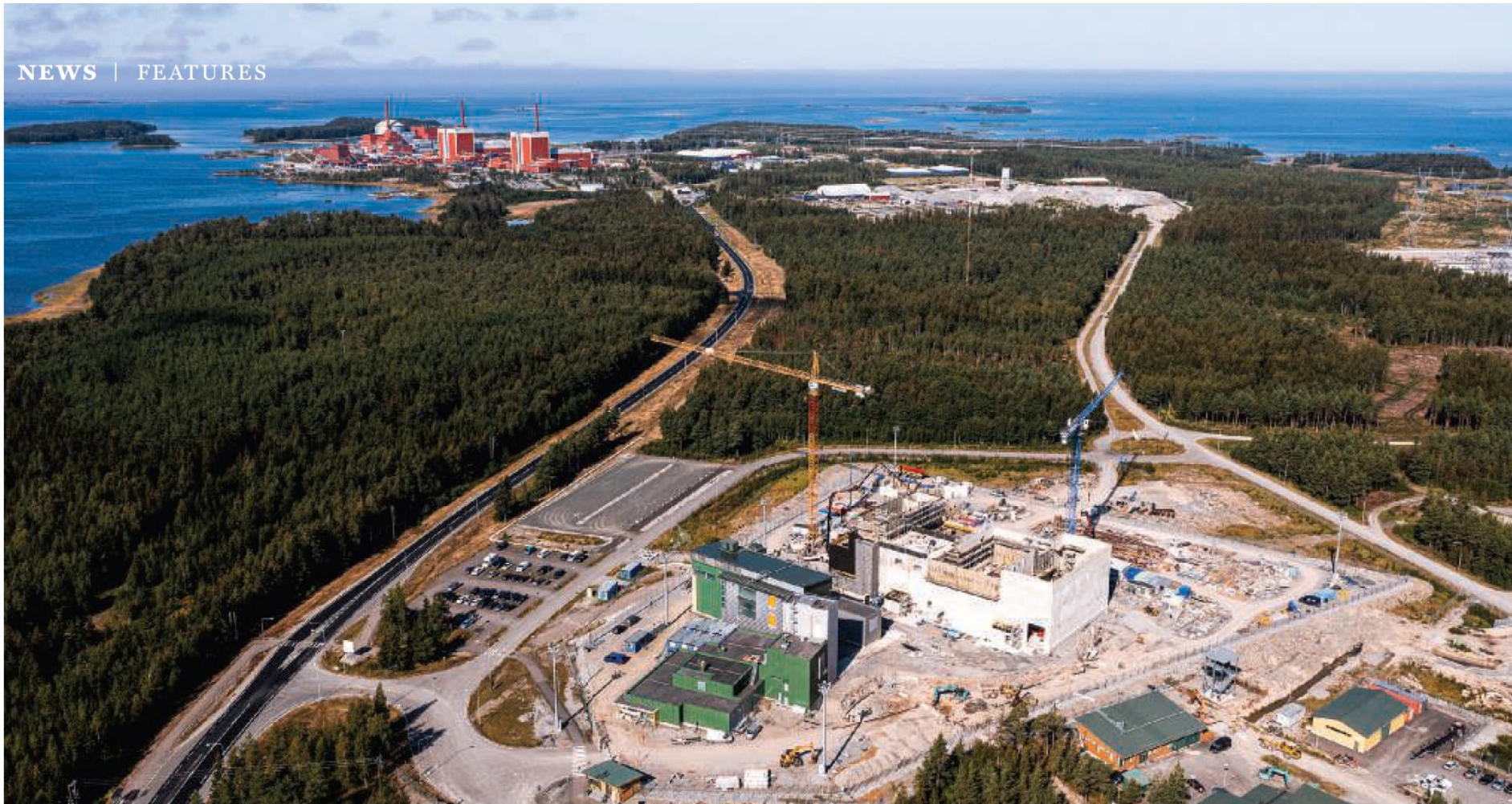
Onkalo's encapsulation plant (white) sits atop an ant's nest of underground tunnels in this August 2021 photo. Olkiluoto's nuclear power plants can be seen in the distance.
